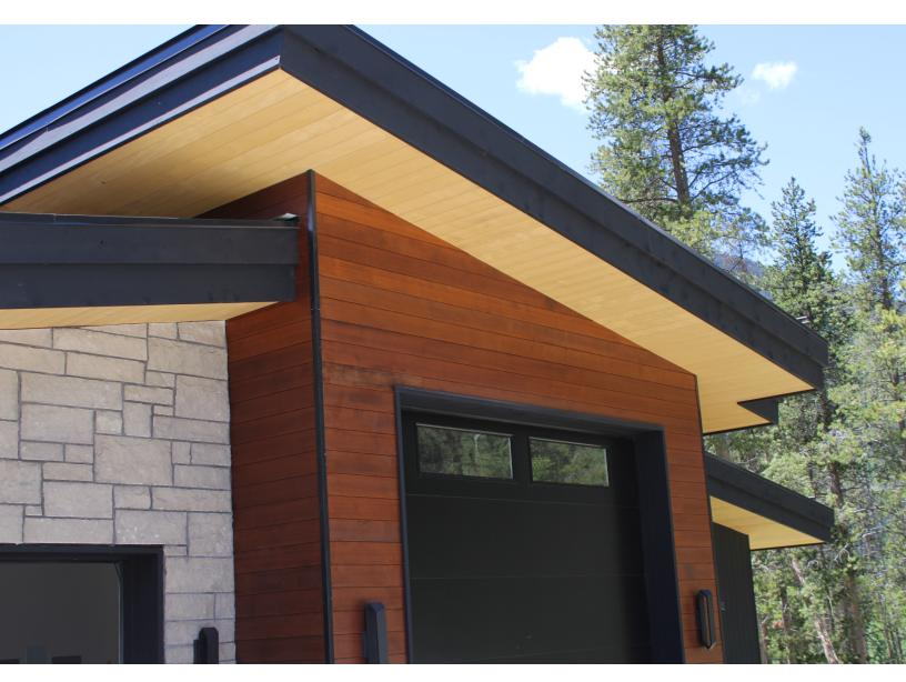
New Age Thermally Modified Hemlock is an all natural building material produced and manufactured in the USA. Thermal modification uses high heat to remove organic compounds from the wood cells. The result is a wood product that does not absorb moisture, expand, contract, warp or become a food source for insects. This process allows you to enjoy the beauty of natural wood in both interior and exterior applications without the worry of rot, decay or harmful chemicals.
