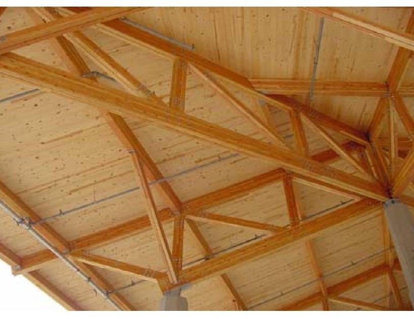
Lock-Deck is a structurally engineered product of two to five kiln-dried lumber laminations bonded together with an exterior waterproof adhesive to form glue-laminated decking. It is commonly used in Heavy Timber construction as well as wood frame and hybrid systems.
